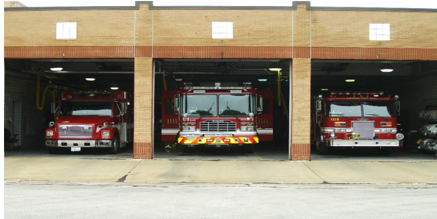
Above is our fire station located at 300 W. Burlington Avenue. Apparatus 'at the ready' to serve and protect the citizens of La Grange.
